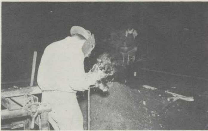
Welding pipes and fittings for plumbing.
