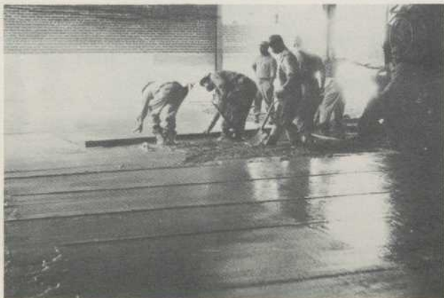
Pouring the cement floor.
