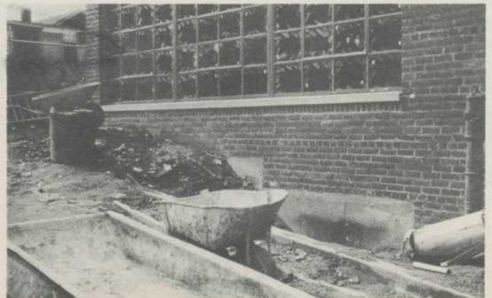
Putting in outside windows.
