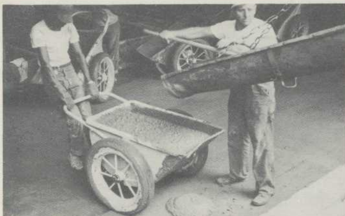
Hauling cement for floors.
