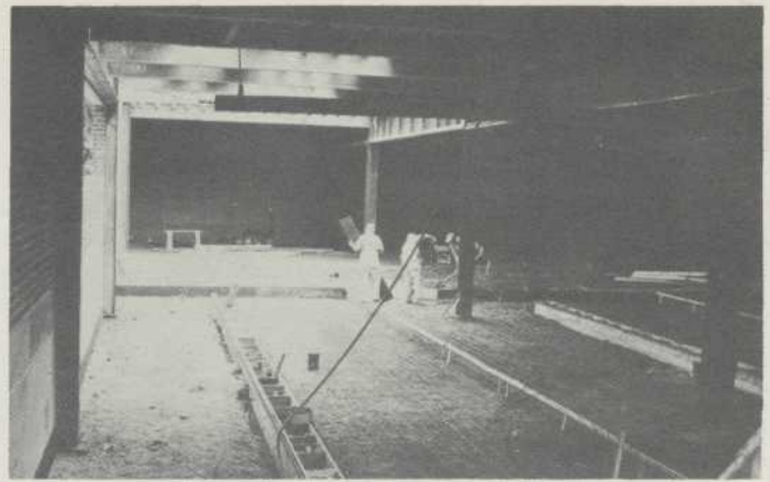
Foundation for future grinding and polishing machines.
