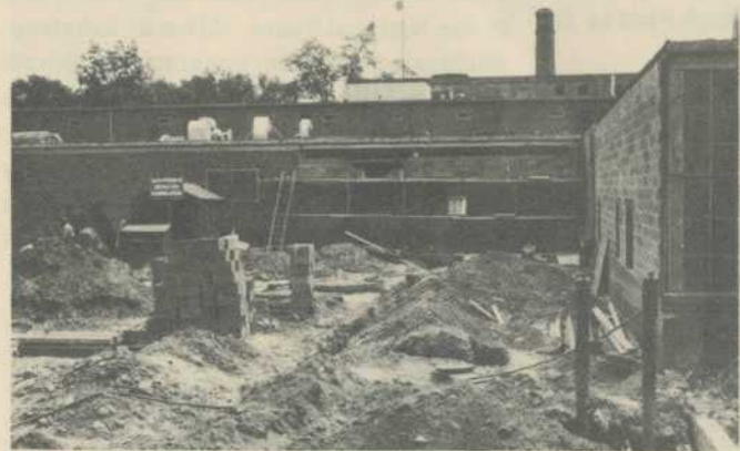
Windows of Plant II become solid walls.
