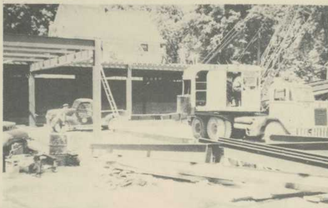
Steel construction starts.
