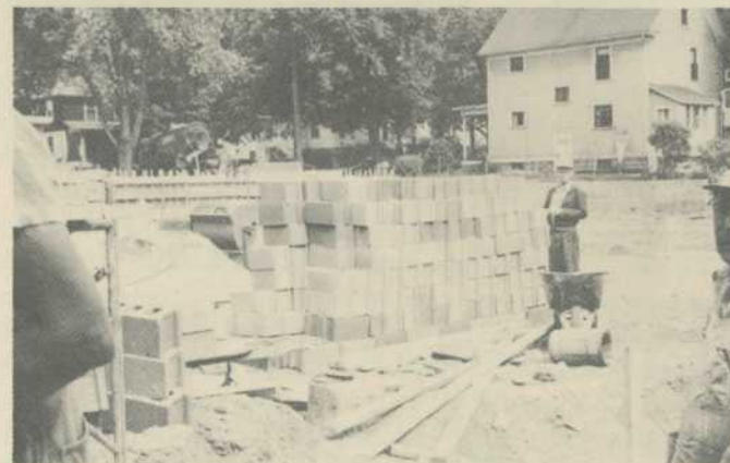
Foundation being laid.
