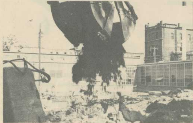
Steam shovel operations begin.
