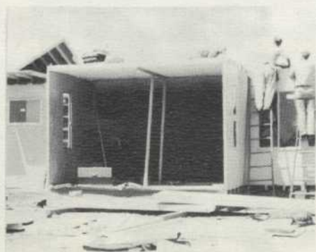
11:00 a.m. The insulation and roofing is installed.
