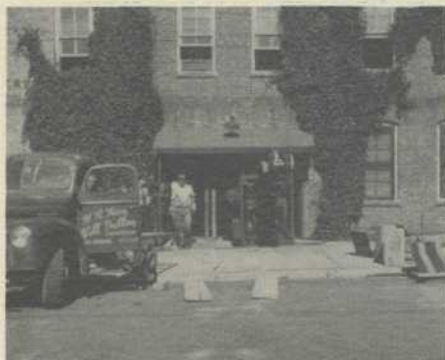
The rig starts through the door.
